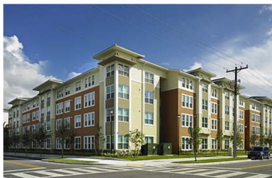
Conventional multifamily construction. Photo courtesy of First Florida Contractors
