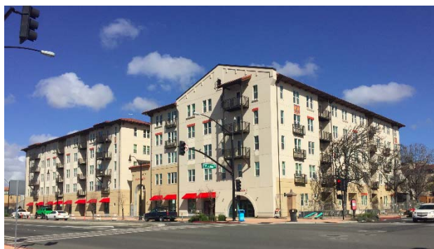
Off-site multifamily construction. Photo courtesy of BRIDGE
