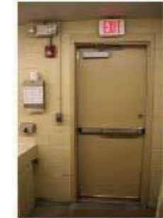
Proper egress door with emergency lighting, signage and panic hardware.
