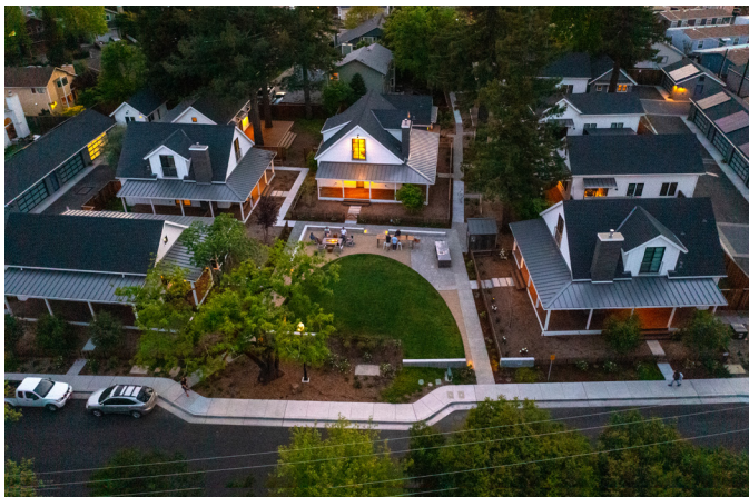
A twelve-unit project in Healdsburg, photo courtesy of Jim Heid.
