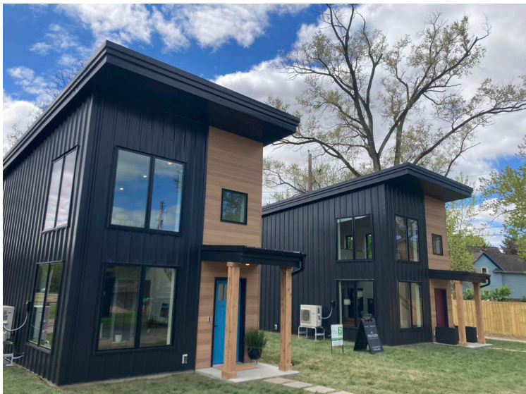
A two-unit project in South Bend, photo courtesy of Mike Keen.
